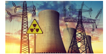
Nuclear power stations
